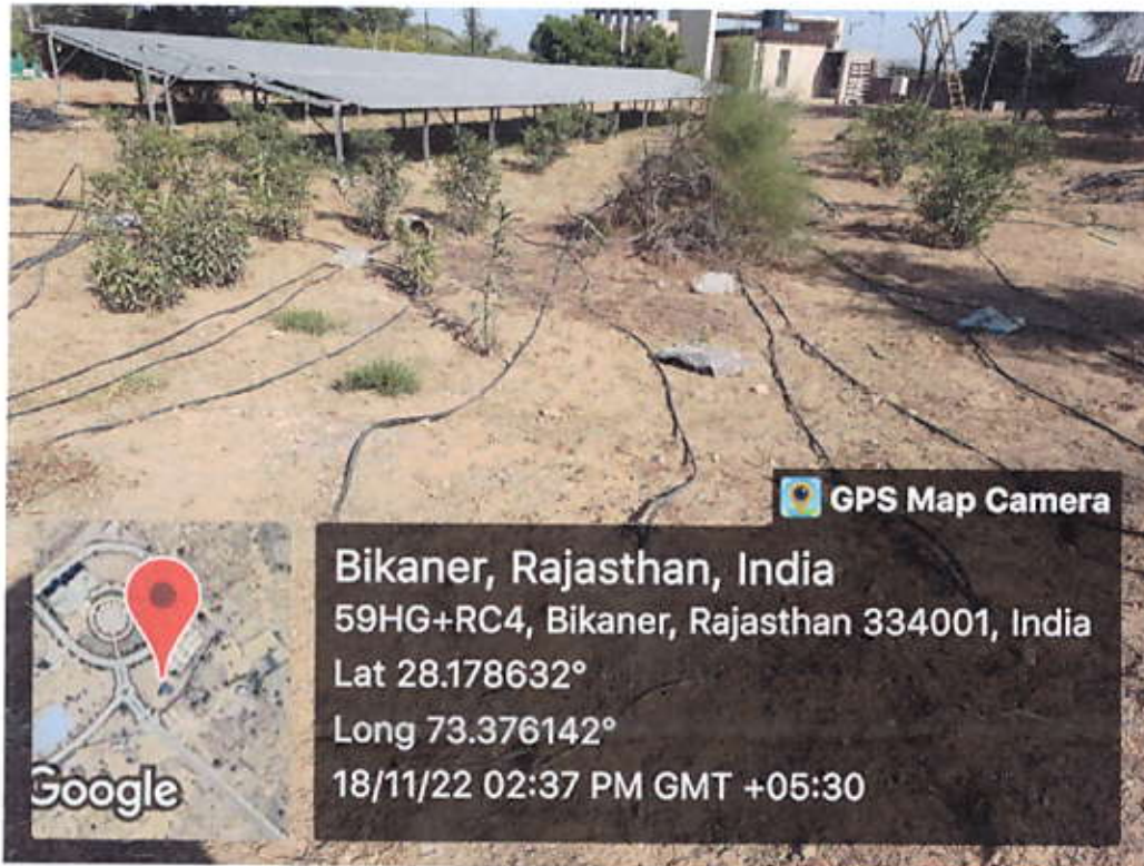
Drip Irrigation System
